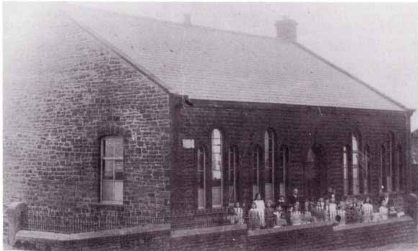
Belthorn and Yate Bank Independent Chapel School. Originally day, evening and Sunday schools were held under the gallery of the chapel but in 1874 land was purchased for the erection of a separate building. The foundation stone was laid on the 8th July, 1876, by the daughter of the Rev. J. H. Unwin. Following the closure of the school in 1966 the building was used for various functions until its demolition. A bungalow, Chapel House, now stands on the site. The photograph, probably taken in 1918, appears to show all the children who were then attending the school. The headteacher, Mr. Jones, is on the extreme right.
