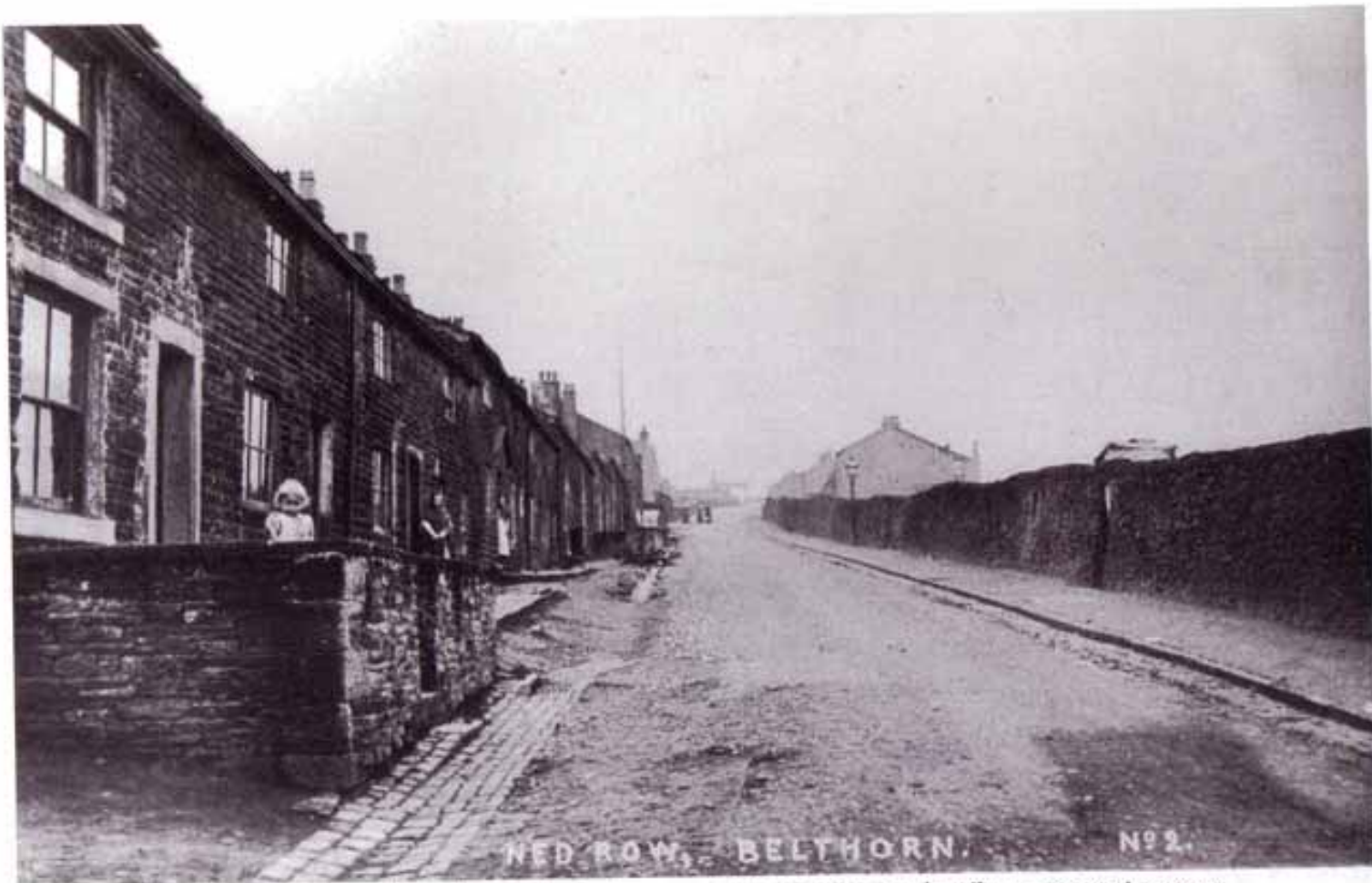
Ned Row, built at the beginning of the nineteenth century, was a terrace of cotton handloom weavers' cottages. The loomshops of each cottage, designed to hold four handlooms, were lit by a pair of windows at ground floor level. By the time this photograph was taken the loomshop of the lowest house had been converted into a separate dwelling. Although one of the windows has been enlarged to form a door, the relationship between the bedroom window and the ground floor openings survived.
